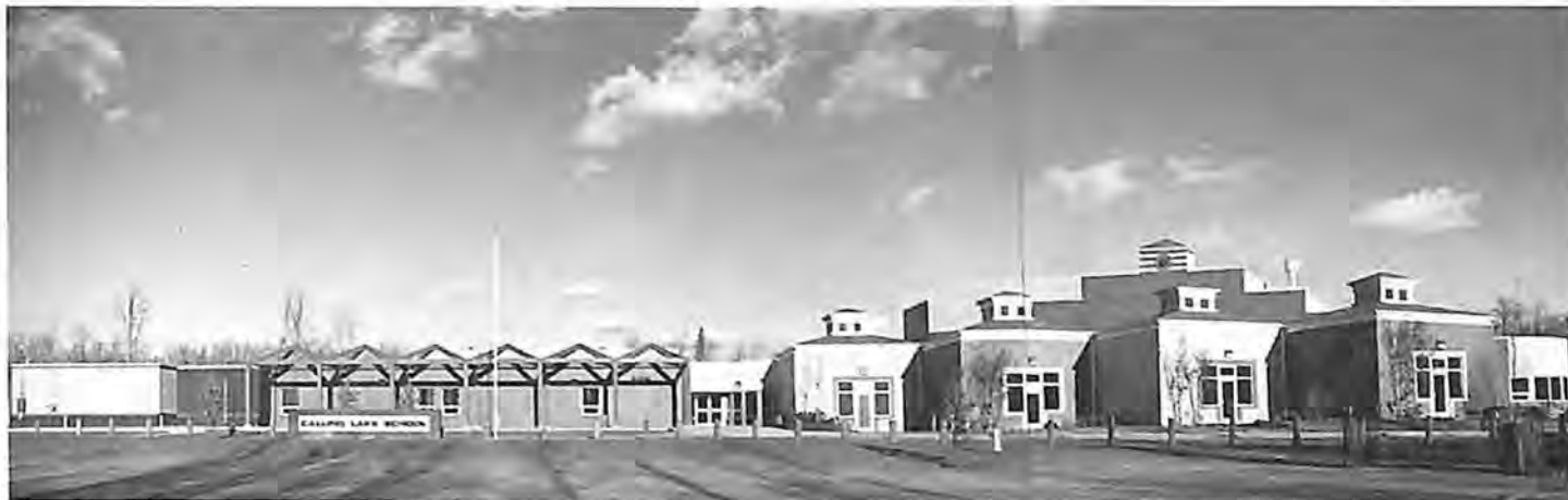
The "new" Calling Lake School Complex, August, 1989.
