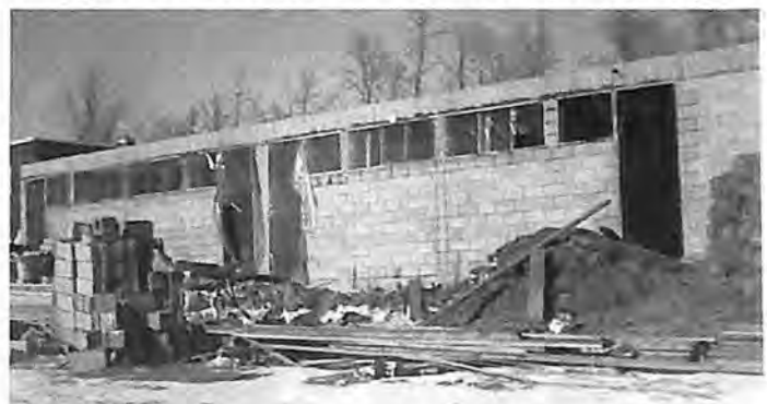
Construction of the cement block addition - photo courtesy EVERGREEN 1967 - 68
