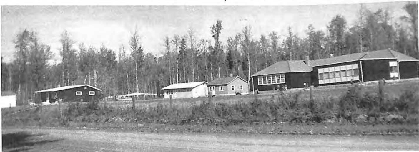
School buildings at Calling Lake, 1963. L-R: Garage, brown teacherage (Yoder), turquoise teacherage (Kornelsen), gray teacherage (Shwaga), four-room school. - photo courtesy Dora Shwaga
