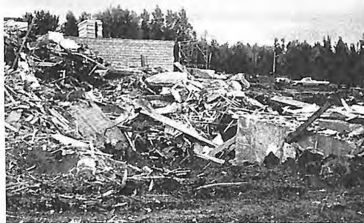
Calling Lake School classrooms, built in 1962 and earlier, were demolished.
